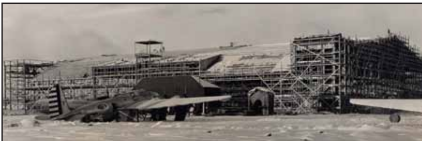
Ladd Field, near Fairbanks, Alaska, was still under construction when the first aircraft arrived. Old Seventy is visible on the right. Sister ship 38-216 is visible on the left. Wings are covered with light cotton cloth to prevent ice buildup.
