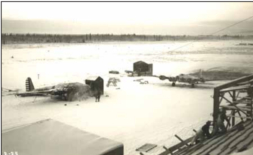
Old Seventy on the left while undergoing engine maintenance. Note the portable shed over a port engine.
